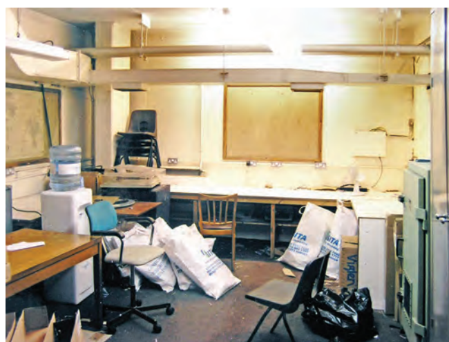
The former communications room in the control centre under Woodville Halls in 1991
